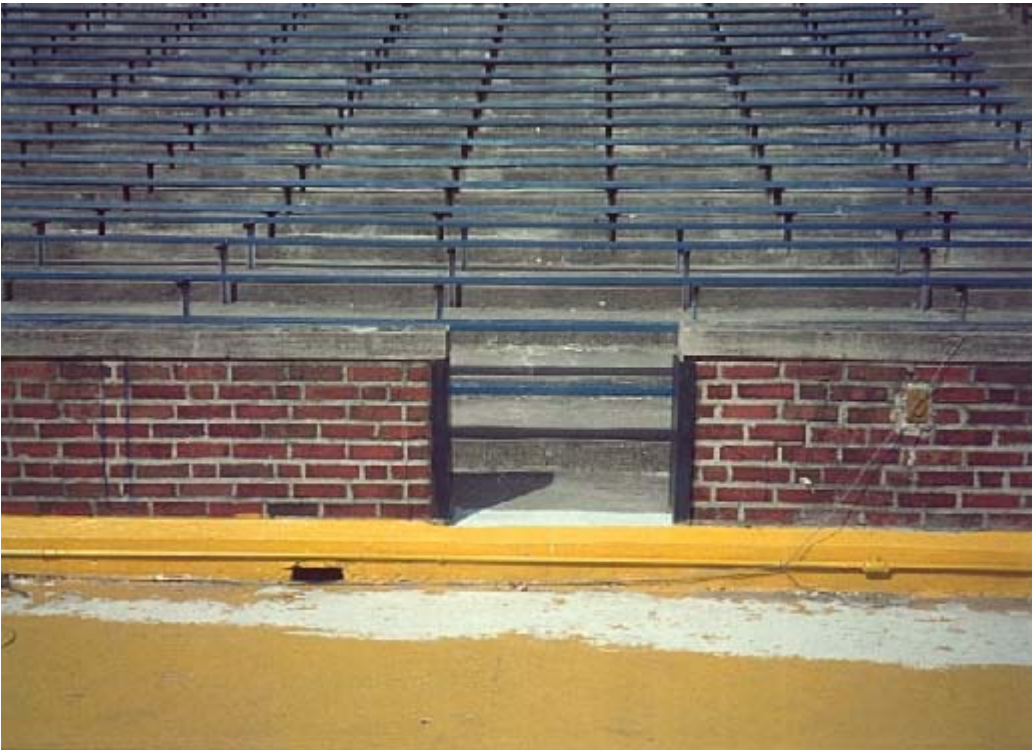
Photograph taken circa 1989. Same location after repair completed.
