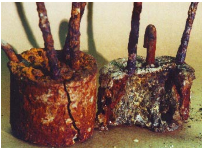
Figure 2. Photograph of IPANEX concrete [left] and the control concrete [right].
